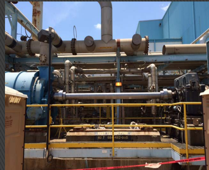
T-FLEX T-9 13 Foot Floating shaft that ATRA-FLEX RUSHED delivery on in 2016 for Domtar in Ashdown, Arkansas. The actual shaft section on this one is 3/4" wall steel tubing.
